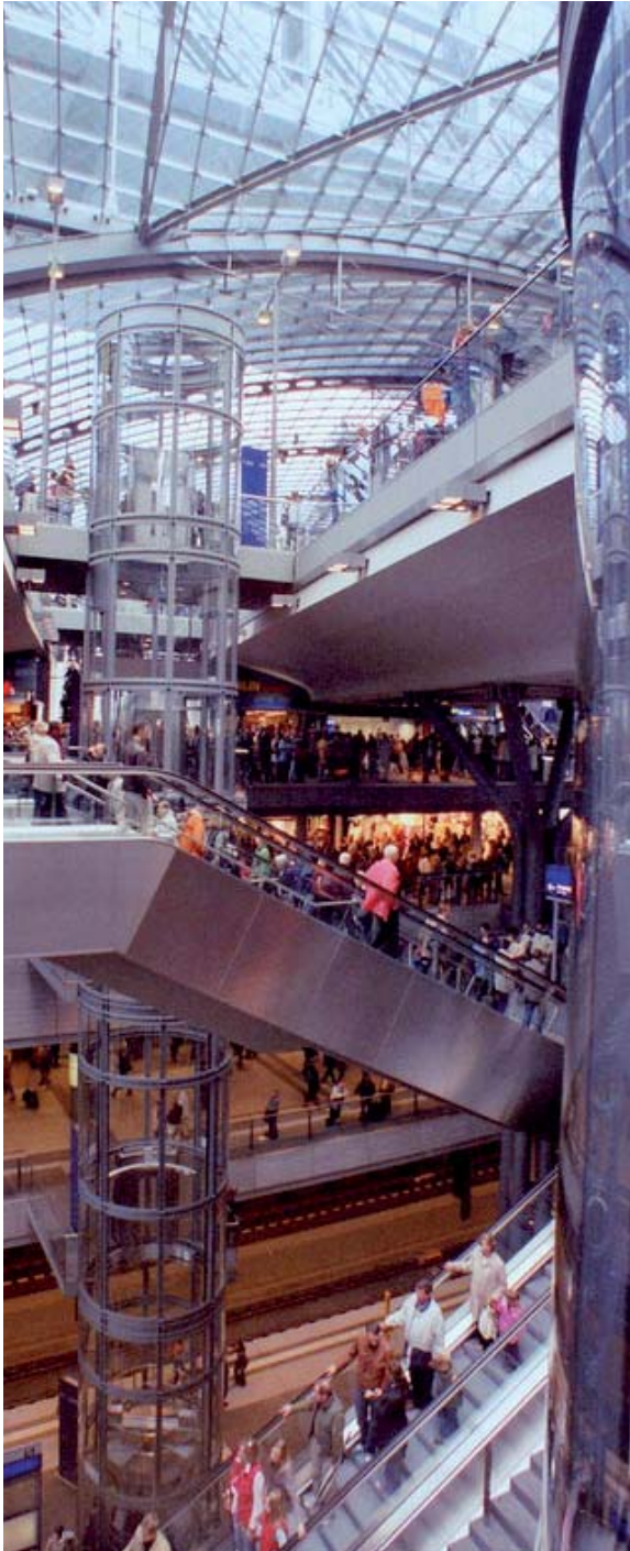
Fig. 25: Hauptbahnhof (main station) in Berlin with escalators and elevators as a design element; by gmp – van Gerkan, Marg und Partner
