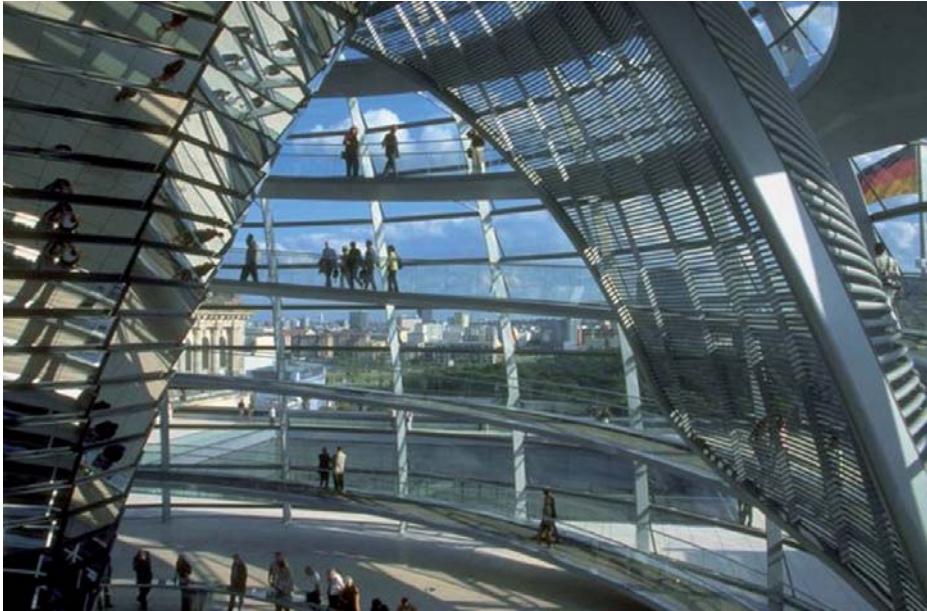
Fig. 21: Dome of the Reichstag by Foster+Partners The ramps are arranged like a winding, so that ascending and descending visitors do not cross one another.
